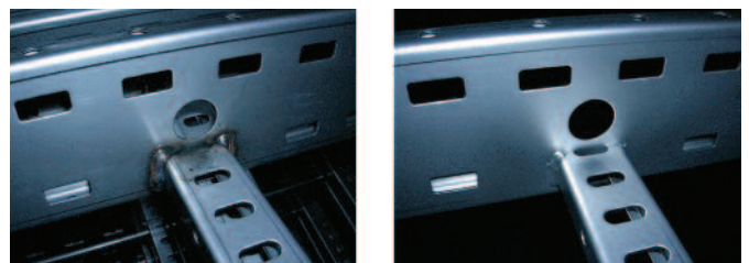
Fig. 10. Stainless steel cable channel treated with water blasting.
